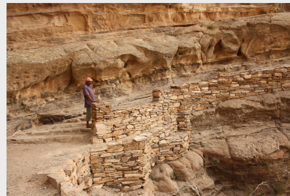
Figure 9. A new trail from Beida area with a local trail guide (photograph by Aylin Orbaşlı, 2015)
