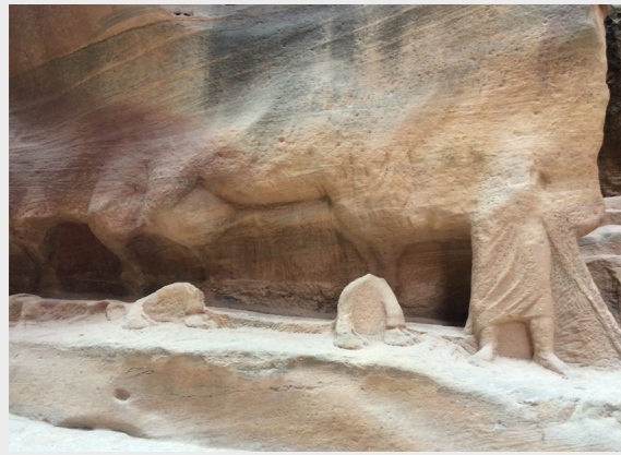
Figure 2. The sandstone is very susceptible to weathering and stone erosion is compounded by flood waters (photograph by Aylin Orbaşlı, 2016)
